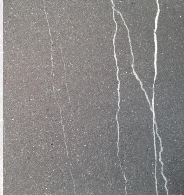
Kalzit-Adern in Bodenplatte
